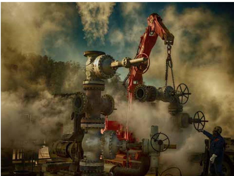
Sartori Fabio Geothermal works 2021
